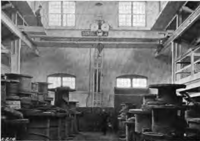
Fig. 1. Floor-operated Traveling Crane, with Foot-Walk and Repair Platform on Girders, Caged Ladders, and Walks Entire Length of Runway over Crane.*
